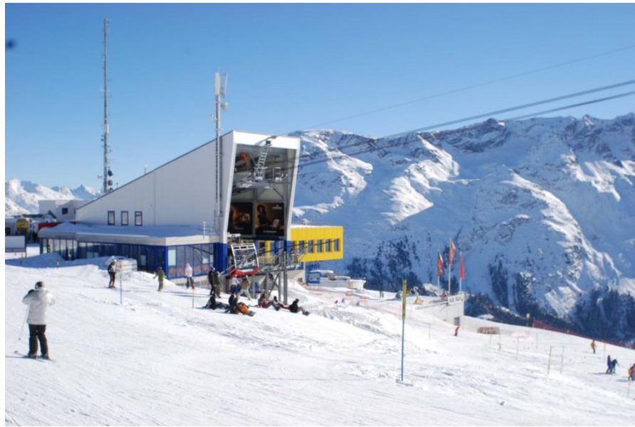
One of the ski lift stations used to reach the top of the St. Moritz – Celerina ski resort pistes.
