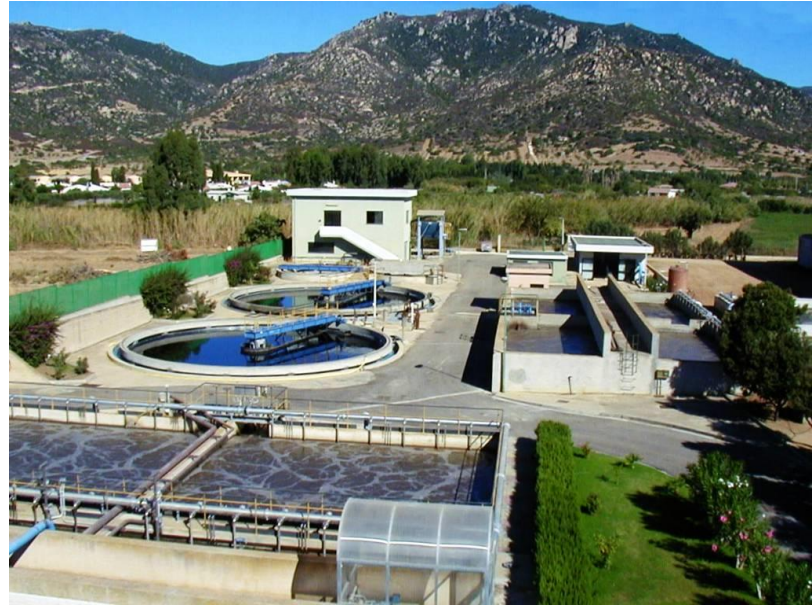
The wastewater treatment process monitored and remote controlled by a system designed by Anova Srl from Naples.
